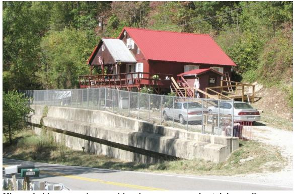
Mine subsidence can be a problem in some areas. A retaining wall was constructed to stabilize the foundation of this home above an abandoned subsiding underground mine in Letcher County. Photo by Dan Carey, Kentucky Geological Survey.
